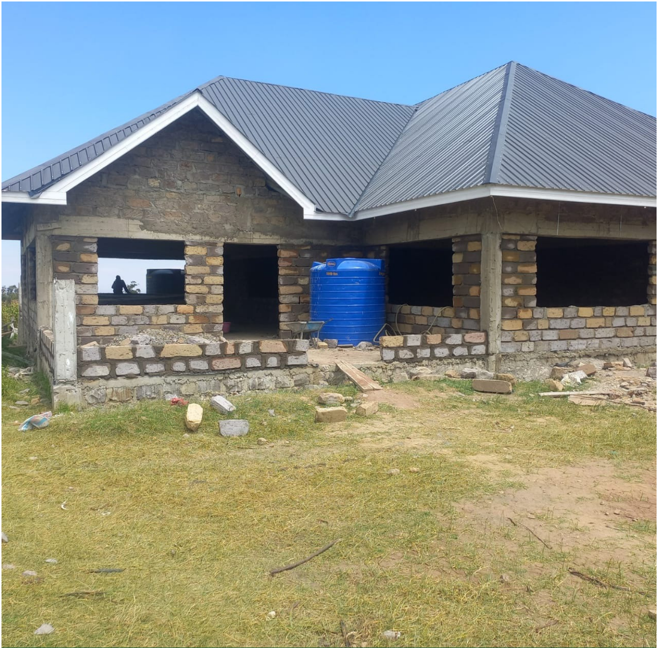
Culture Centre construction in progress.
